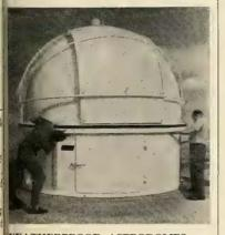
VEATHERPROOF ASTRODOMES are eing used to protect instrumentation, notion picture cameras, telescopes and ther equipment used in tracking missiles. I anufactured by the Houston Fearless Corp., the astrodomes are made of imregnated honeycomb covered with fiber lass.
