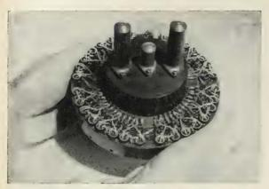
INSTRUMENTS THAT measured the two radiation belts during the flight of Pioneer III on Dec. 6-7. The two Geiger-Mueller tubes measured the intensity levels.
