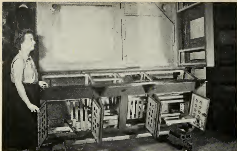
MAGNESIUM FABRICATED radar cabinet for Nike-Ajax weighs only 280 pounds.
