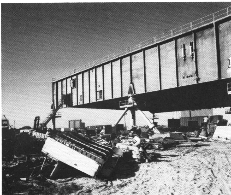
Figure 3 LUT base after removal of tower and Saturn 1B adapter pedestal, November 1983.
