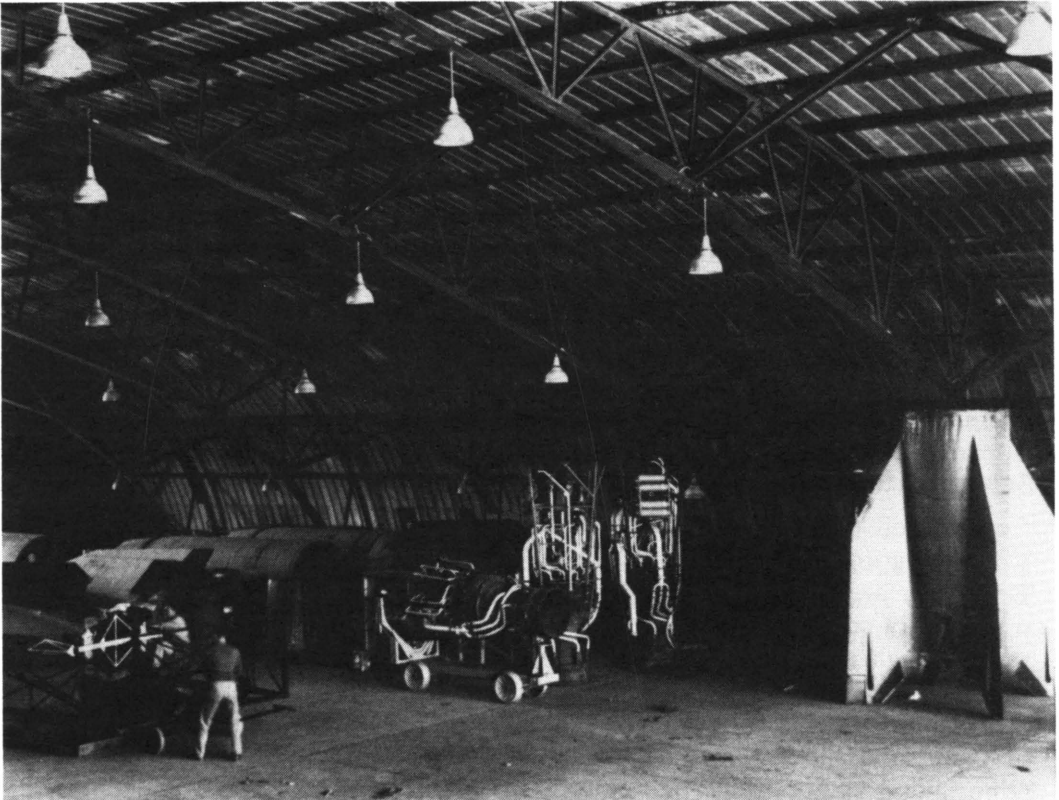
Figure 4 V-2 components in Missile Assembly Building #1.
