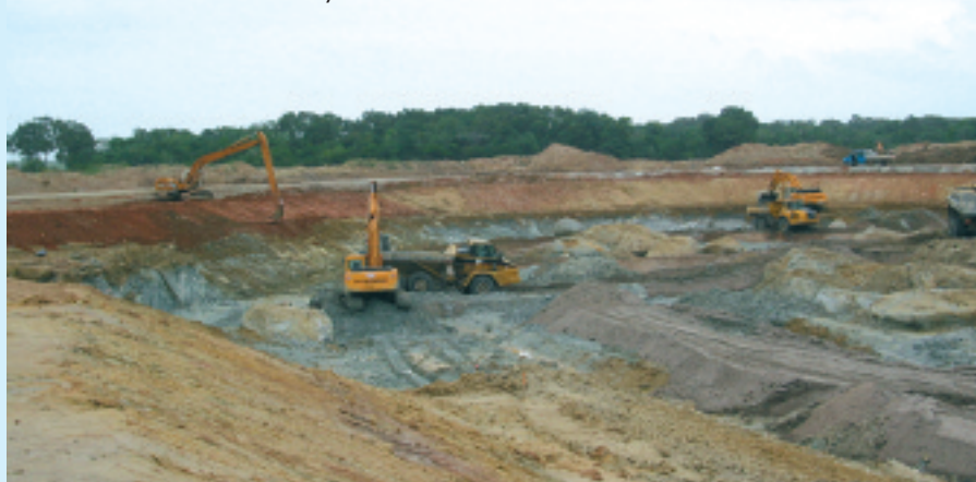
Excavation of the flame chute for the Soyuz Launch Site
