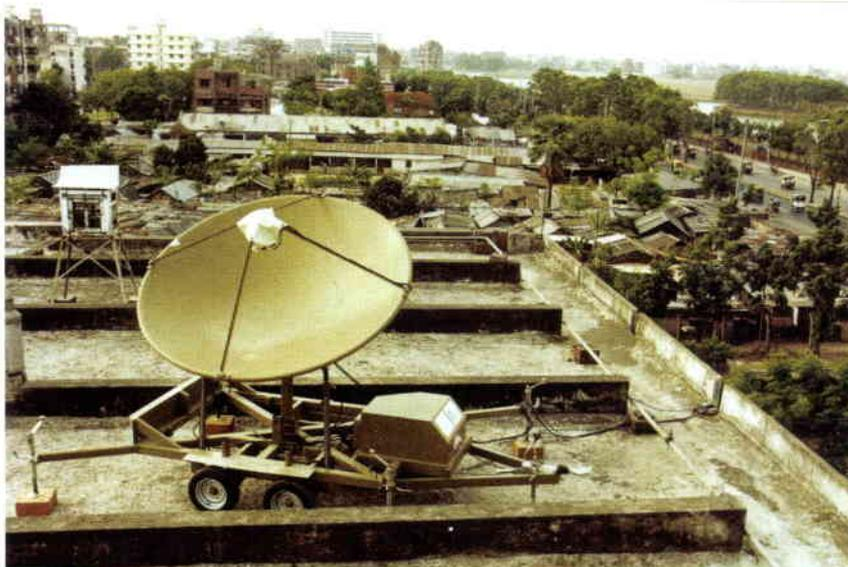
**Figure 10. A RAPIDS mobile station (dish antenna and hydraulic control system) deployed on the roof of SPARSSO agency in Bangladesh**
