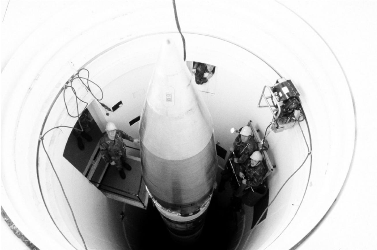
**Minuteman in silo.** Ballistic missile operations moved from above ground sites to underground silos. This Minuteman ICBM silo provides not only environment protection, but secures the missile against a near nuclear explosion. (Courtesy, U.S. Air Force)
