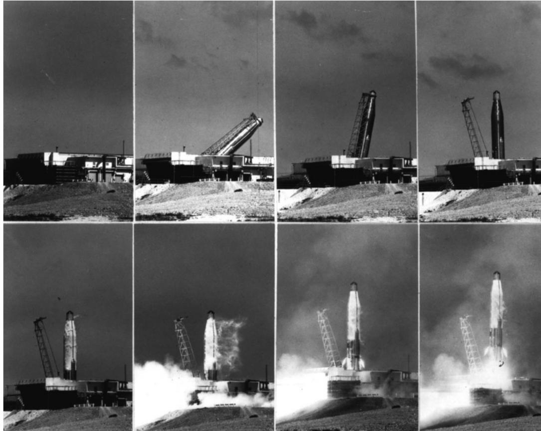
**Atlas launch sequence.** Atlas crews had to lift their weapons from a coffin storage facility into a firing position. These images demonstrate a typical Atlas launch sequence that could take at least fifteen minutes for fueling, guidance, and other operations. (Courtesy, U.S. Air Force)
