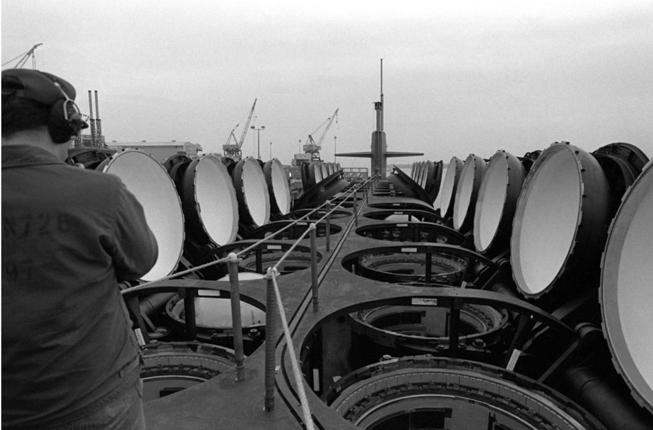
**Ohio SSBN.** Ohio-class SSBNs hold up to twenty-four Trident SLBMs. An internal pressure system allows SSBN crews to push the SLBM through a breakable inner hatch. Once the SLBM breaks the surface, the rocket motors will ignite. (Courtesy, U.S. Navy)
