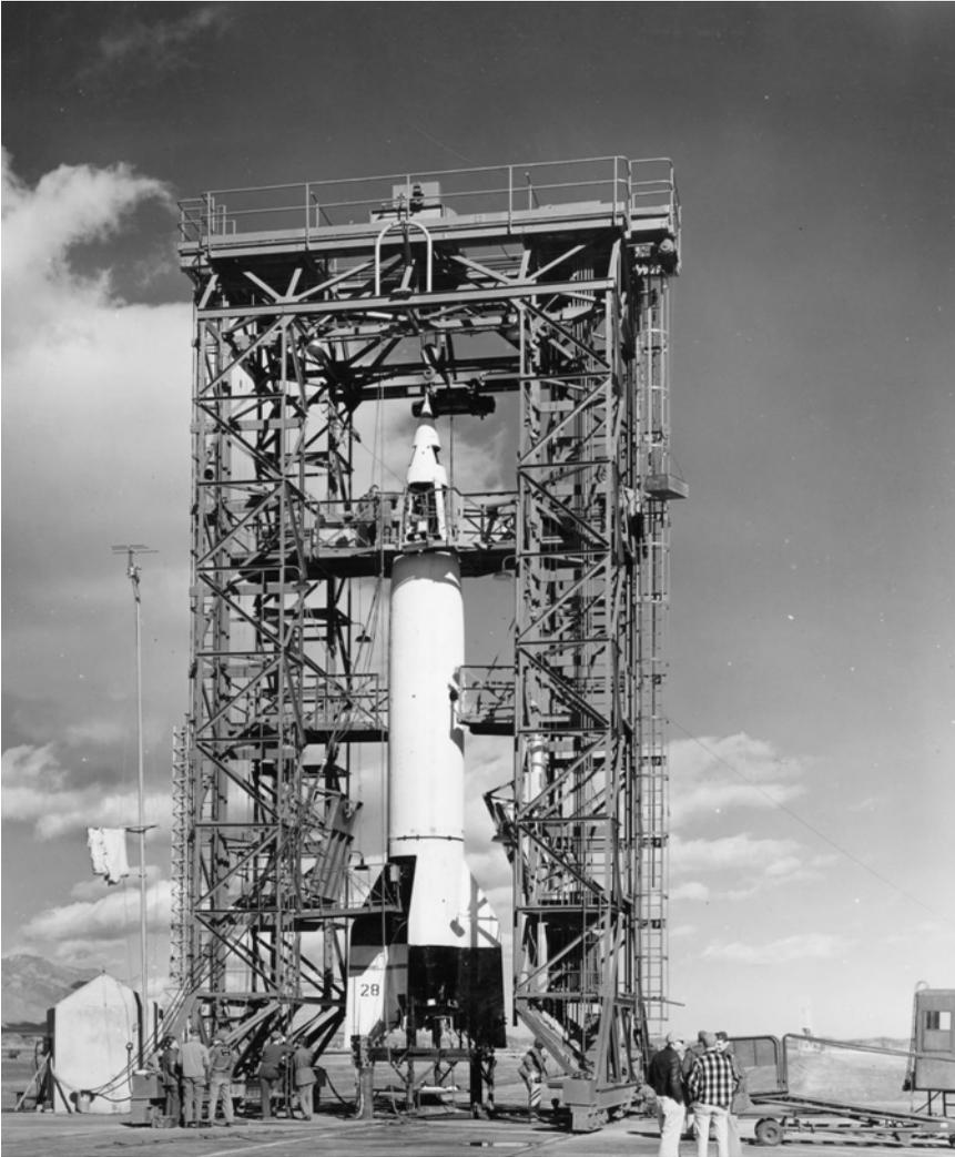
**V-2 on launch pad.** The German V-2 was a key element of early U.S. and Soviet ballistic missile development. This V-2, at White Sands in New Mexico, served as a test bed for the U.S. Army and allowed engineers to experiment with several new technologies. (Courtesy, U.S. Army)
