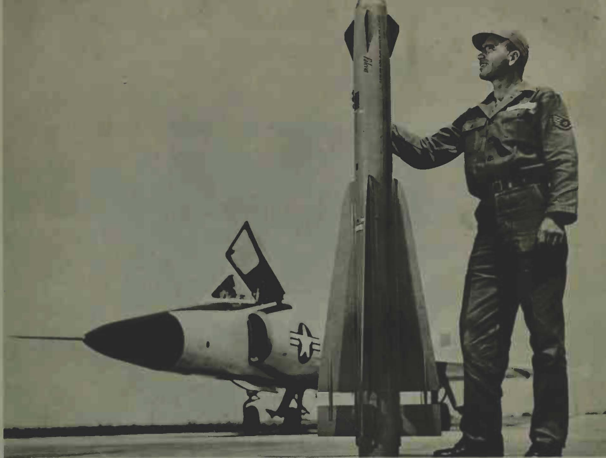
F-102 "Delta Dagger" fighter forms backdrop for Hughes GAR-1D Falcon guided aircraft rocket displayed by an Air Force sergeant. The Falcon's powerplant provides supersonic speed as its own guidance system directs it to a maneuvering target.
