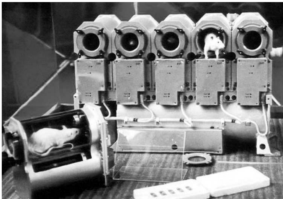
The rat cages for Cosmos 782, consisting of individual cylinders for the rats, with waste collection below. This hardware was used on the first four collaborative Bion flights. (Photo: Dr. Delbert Philpott, courtesy NASA Ames History Office)
