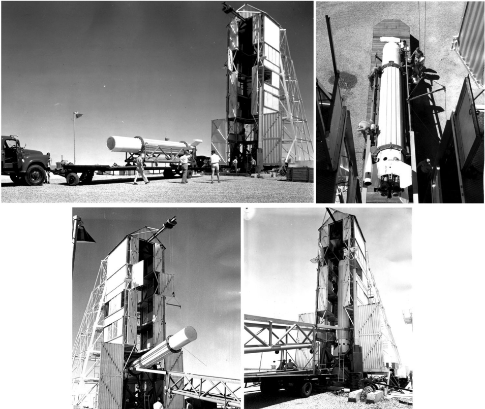
Figure 84. An early non flight vehicle being used to test out the gantry at Woomera. This was a thin walled stringered version which was not put into production.
