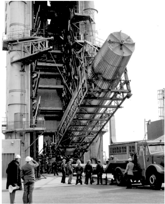
Figure 44. An early test vehicle being lifted up into the stand at the de Havilland factory at Hatfield.
