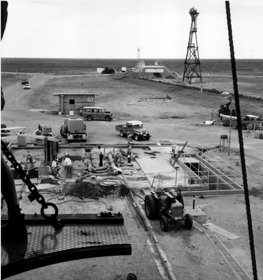
Figure 113. One of the two Black Knight gantries was rebuilt for Black Arrow. In the distance is the equipment centre, from where the launches were controlled.
