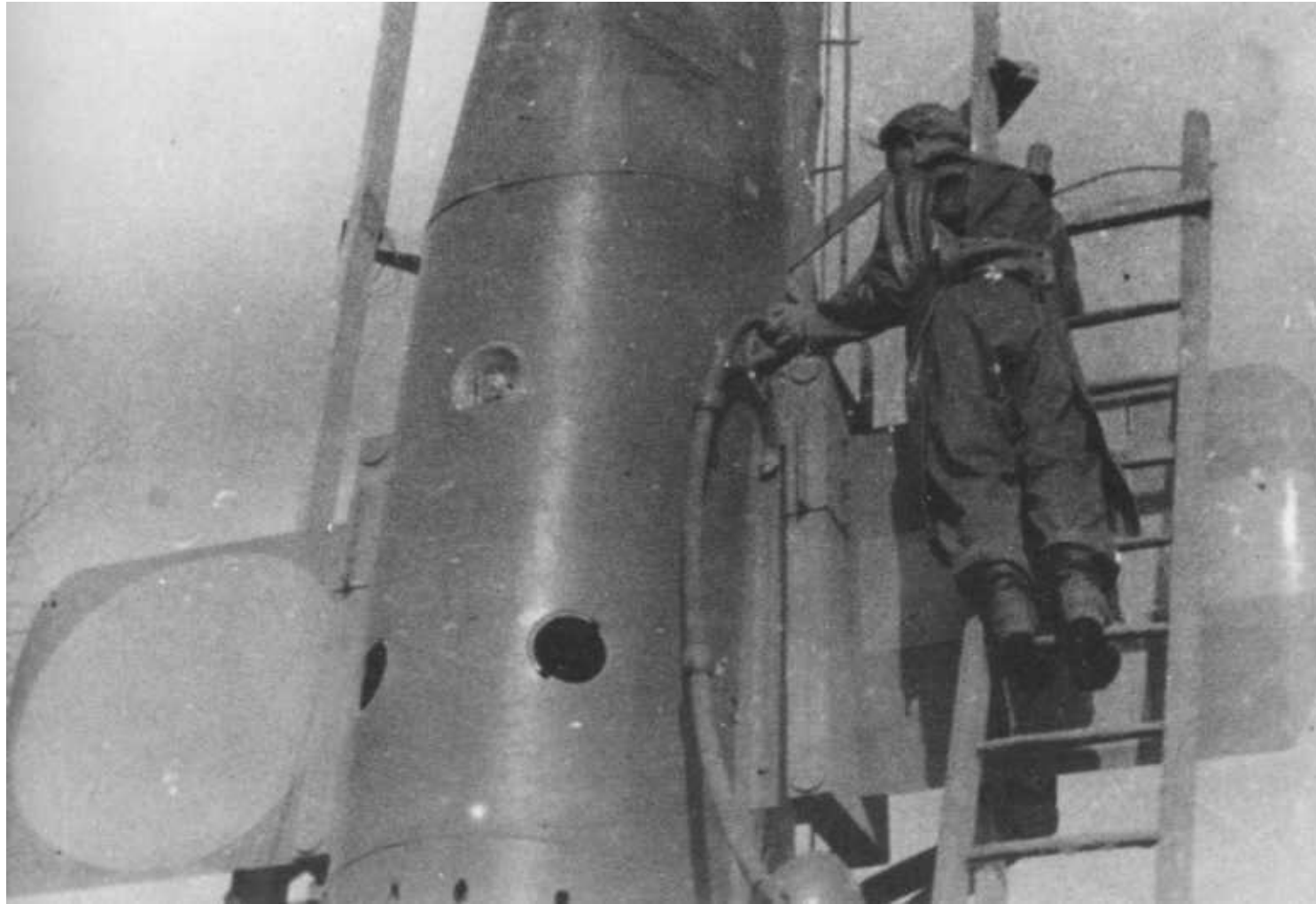
A Bachem Werke HWK 509 specialist is refueling a "Natter's" C-Stoff tank. This tank held approximately 66 gallons [270 liters]. Notice the protective outer clothing the man is wearing. This Ba 349 is mounted on a 70 foot pine tree pole. The refueling filler for the T-Stoff tank can be seen above the two access ports to the HWK 509 mixing motor.
