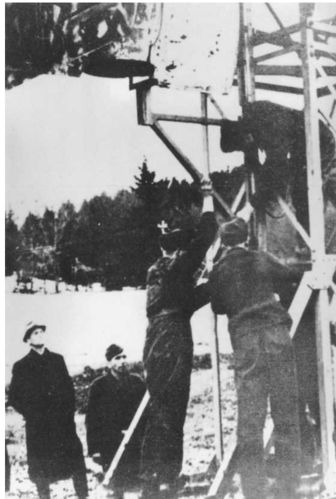
Another 349V as seen above but with a close-up of its tail cone where the HWK 509 would extend out. As many as four Bachem-Werke laborers plus a man in a light-colored hat appear to be concerned with some aspect of the middle launch rail where the 349V's ventral tail rides during lift-off.
