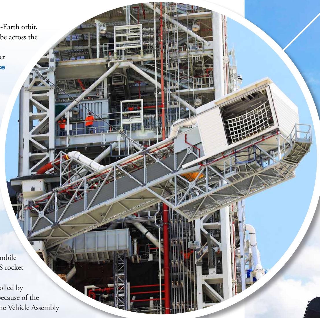
(Above) Technicians and engineers in Exploration Ground Systems at NASA's Kennedy Space Center recently tested the Crew Access Arm that was added on the mobile launcher. The mobile launcher is being prepared to support the agency's Orion spacecraft and Space Launch System rocket. Photo credit: NASA/Kim Shiflett
