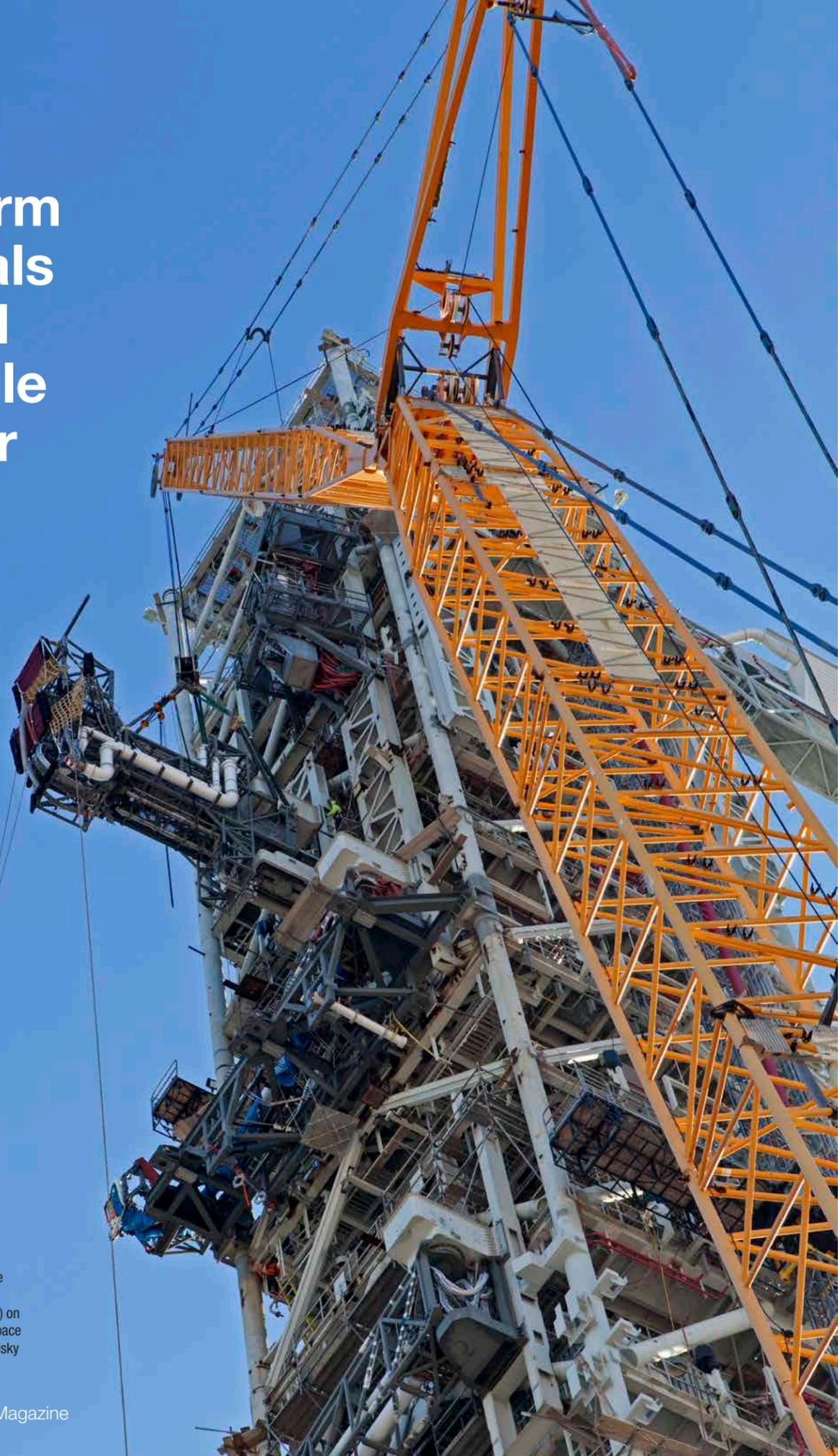
The Interim Cryogenic Propulsion Stage Umbilical (ICPSU) is lifted high up for installation on the mobile launcher (ML) on March 16, 2018, at NASA's Kennedy Space Center. Photo credit: NASA/Ben Smegelsky
