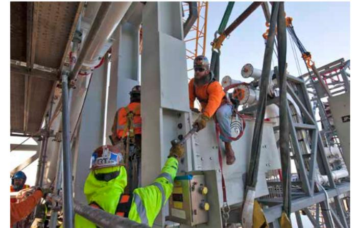
Construction workers with JP Donovan install the Interim Cryogenic Propulsion Stage Umbilical (ICPSU) to the tower of the mobile launcher at about the 240-foot-level on March 16, 2018. The last of the large umbilicals to be installed on the tower, the ICPSU will provide super-cooled hydrogen and liquid oxygen to the Space Launch System rocket's interim cryogenic propulsion stage, or upper stage, at T-0 for Exploration Mission-1. Photo credit: NASA/Ben Smegelsky
