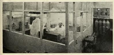
"Clean room"—working areas with controlled, dust-free atmospheres—aren't limited to the guidance manufacturers. The Superior Valve and Fittings Co. of Pittsburgh recently placed in operation a 16 x 16 ft. room for processing precision valves and parts for missiles.
