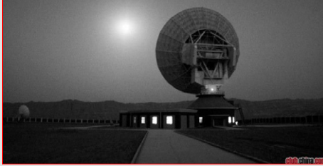
The 35 m diameter antenna in Kashi. Equipped with the S/X/Ka tri-band system, it was also completed in 2012 and supported the Chang'e 2 extended mission and follow-on lunar missions. (credit: China.com)
