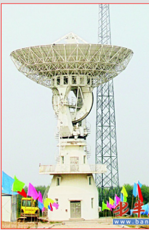
The 18 m diameter antenna in Qingdao tracking station. This antenna, together with the same type of antenna in Kashi, was completed in 2007 to support the Chang'e 1 lunar mission. They are for the first time equipped with an X-band telemetry, tracking and communication system and were tested during the Chang'e 1 mission. These two 18 m antennae built the foundation for China's deep-space tracking network established thereafter. (credit: Bando.cn)
