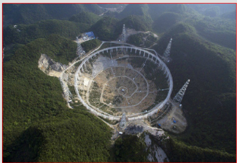
FAST in construction. This photo was taken in early 2015 when its circular girder, six feed towers and the flexible net under the reflector surface had been completed. On 2 August 2015, the first of the 4,450 adjustable reflector panels was installed. (credit: Chinese internet)
