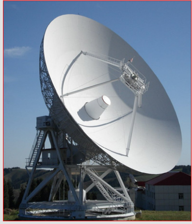
The 66 m diameter antenna in Jiamusi after completion. As the backbone of China's deep-space network, it supported the Chang'e 2 extended mission (EM-L2 point orbiting and Toutatis fly-by), Chang'e 3 and the Chang'e 5-T1 missions. In June 2015, it captured signals from the New Horizons Pluto probe from 4.76 billion kilometres away from the Earth. (credit: Chinese internet)
