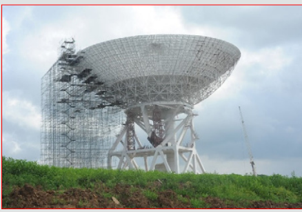
The 66 m diameter antenna under construction in Jiamusi. China began building its own deep-space tracking network after the Chang'e 1 mission. The network includes three stations in Jiamusi, Kashi and Nuequen, Argentina. The Jiamusi antenna, with support of S/X bands, was completed in 2012 and is the largest antenna in China. (credit: Chinese internet)
