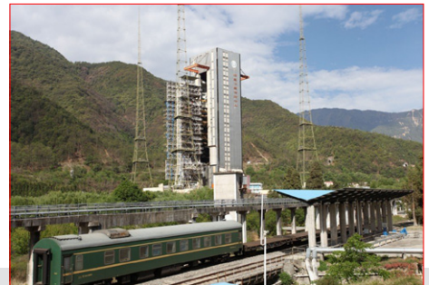
The railway terminal near the launch pad. Pad 2 and the abandoned railway and tunnel to the unbuilt manned launch pad, Pad 1, can also be seen. (credit: Chinese internet)
