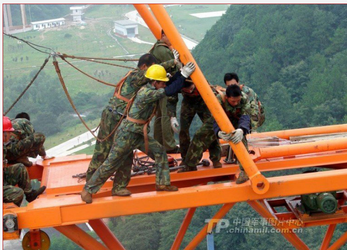
Construction of the new tower of the Pad 3 (credit: Chinamil.com)
