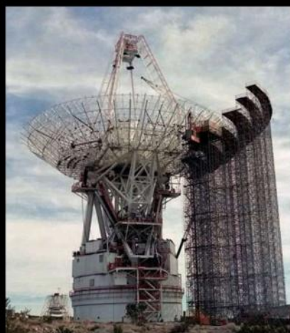
△ The DSS-14 antenna at Goldstone was widened from 64m to 70m in 1989 to help it pick up Voyager 2's weakening signal
