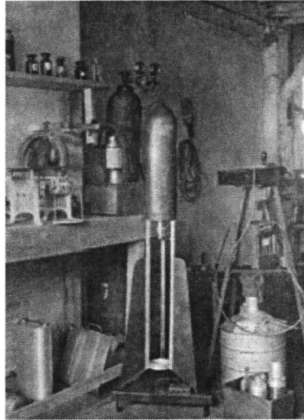
Figure 12–6: New Version of HW1 with fins.
