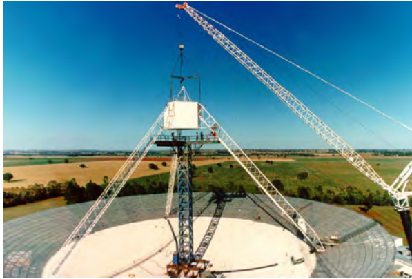
Figure 14–8: Installation of the NASA-funded enlarged focus cabin on the Parkes telescope. This enabled Parkes to support the Galileo mission at Jupiter, while still undertaking its regular radio astronomy observation program. Credit: CSIRO.
