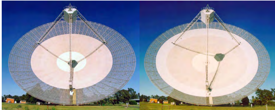
Figure 14–9: Before and after comparison of the upgrade to the Parkes antenna in 2003, showing the additional aluminum paneling added to increase the dish’s sensitivity to X-band signals. Credit: CSIRO.
